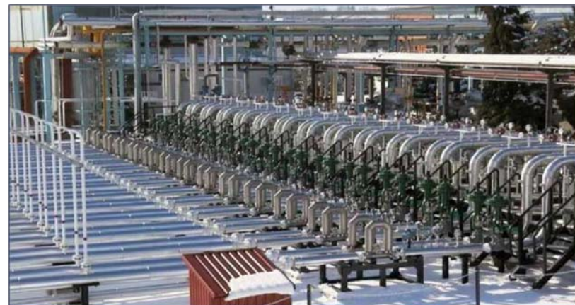
Natural Gas Cavern Storage
